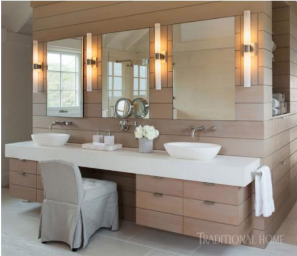
Bathroom floors, walls, and vessel sinks are limestone.
